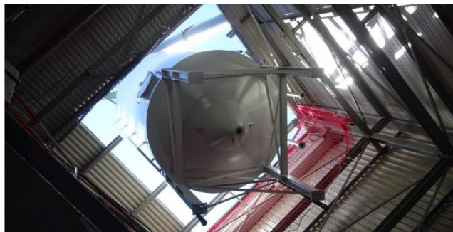
Lifting of the AirPrex® Reactor
